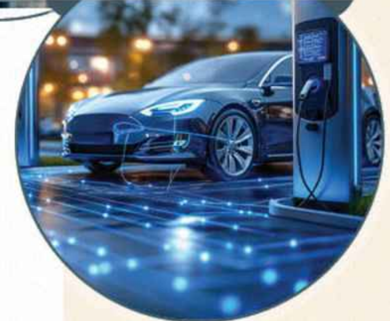
E.V. Charging Point
